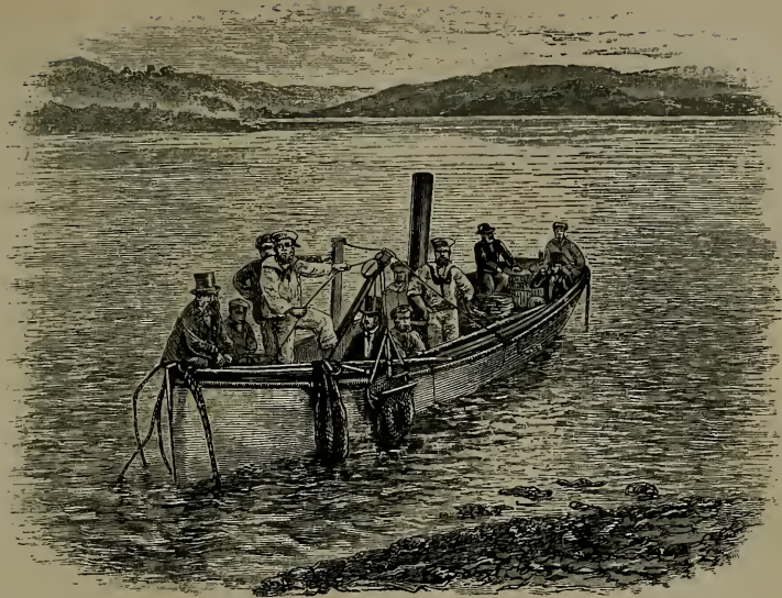
DREDGING ON THE PARAMATTA RIVER, SYDNEY.
